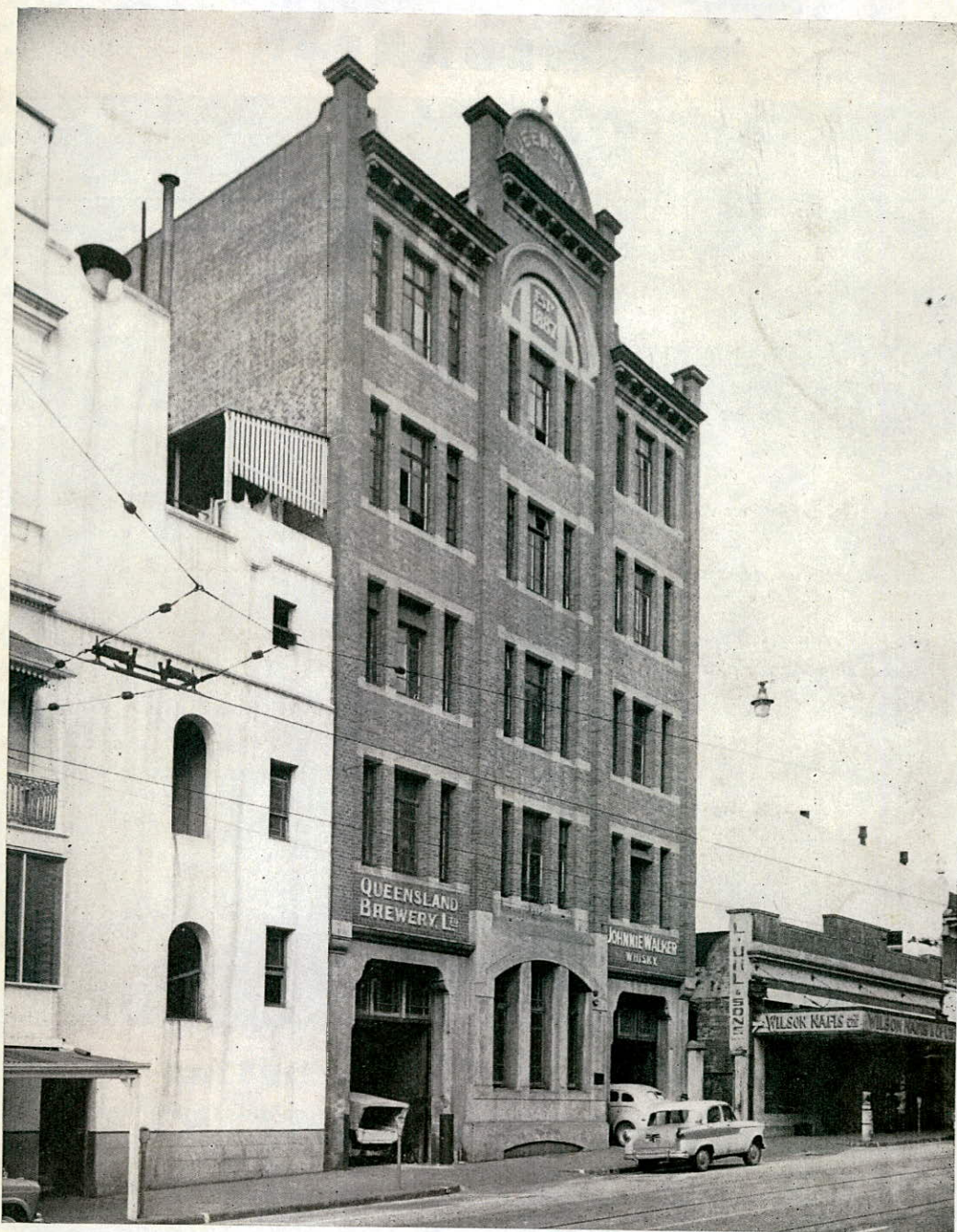
Vacant 5 storey brick building fronting Adelaide Street
