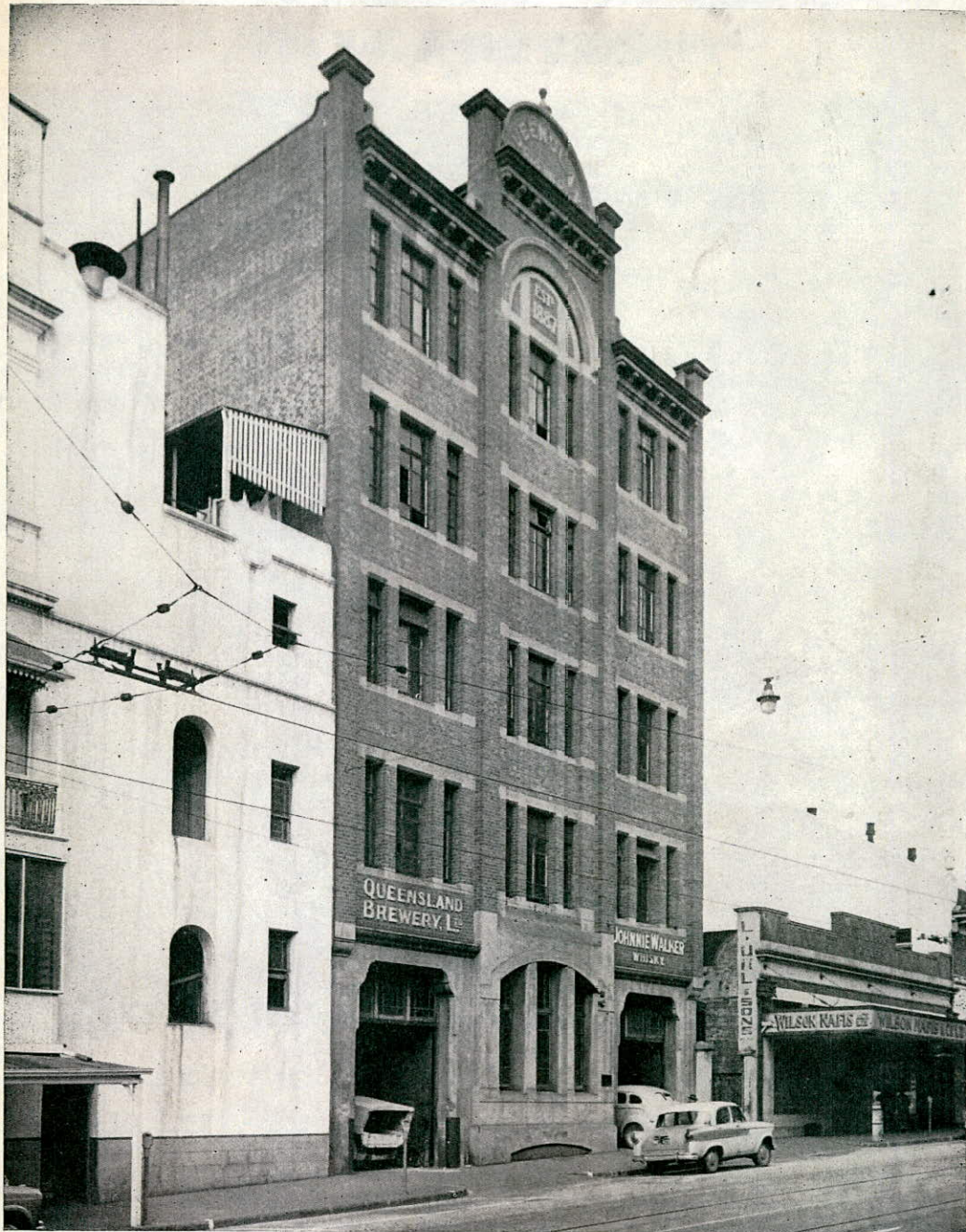
Vacant 5 storey brick building fronting Adelaide Street
