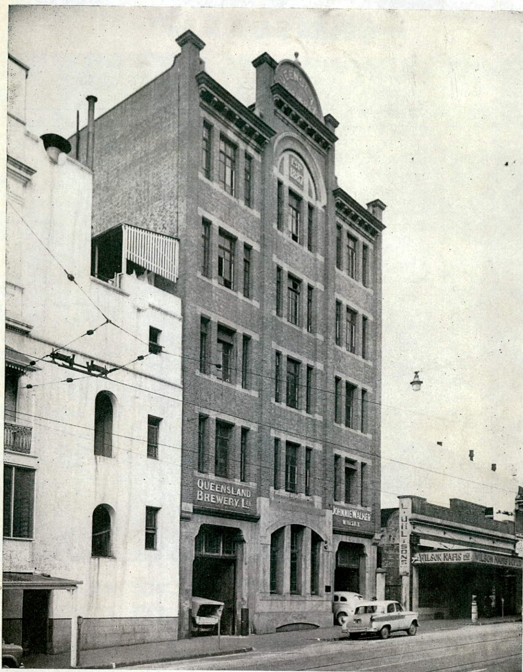
Vacant 5 storey brick building fronting Adelaide Street
