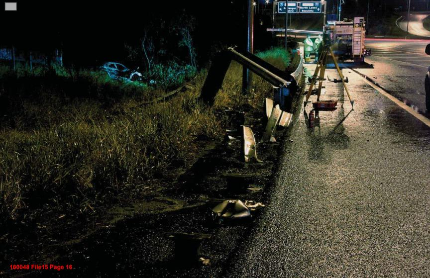
Photograph No. 6: Photograph of the start of the damaged section of w-beam barrier. Visible in this photograph are the commencement of wheel tracks into the grass.
