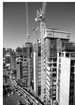
Construction of the new Supreme and District Court complex
