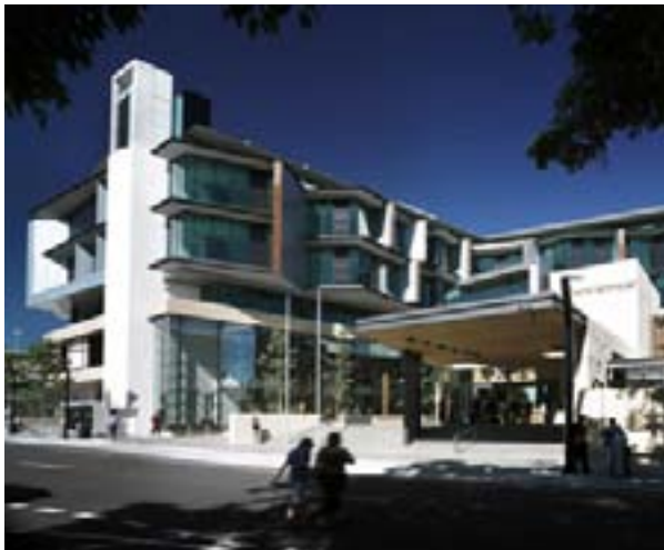
Newly completed Ipswich courthouse and watch house
